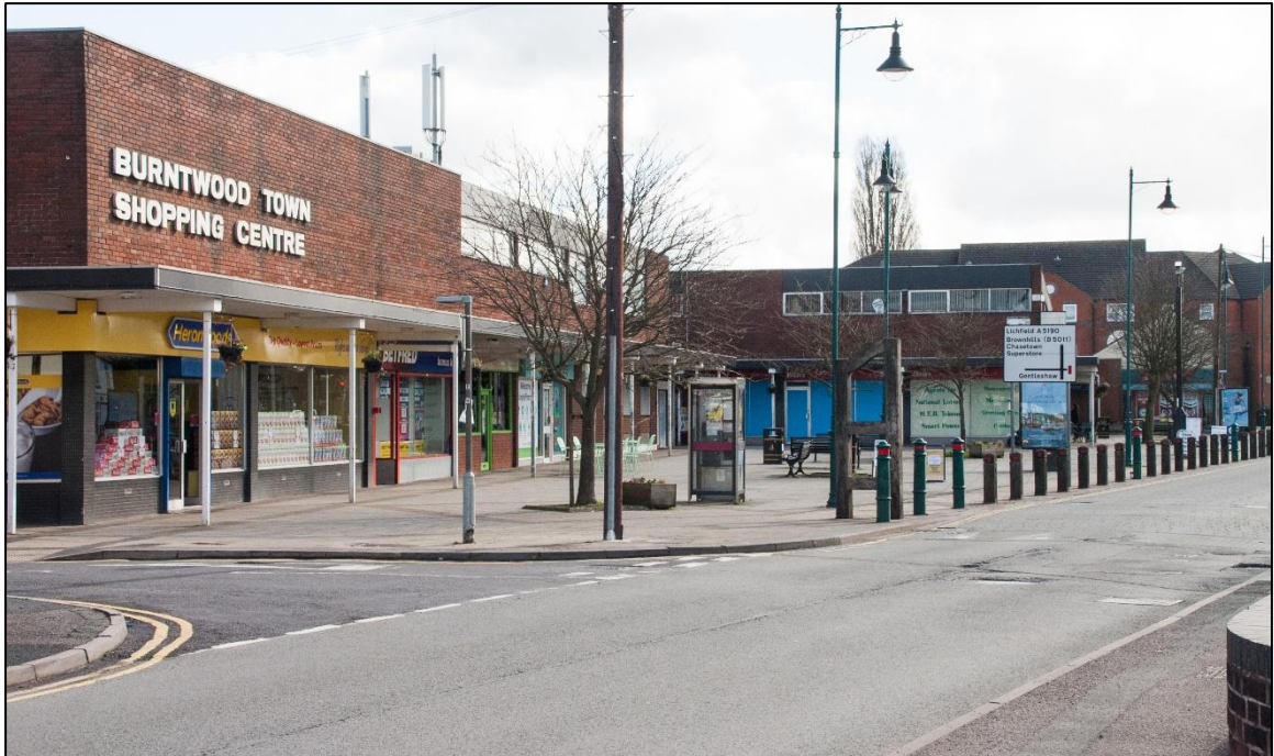
Burntwood Shopping Centre, Sankey's Corner
