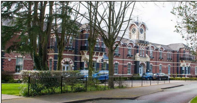
St Matthews Hospital site
