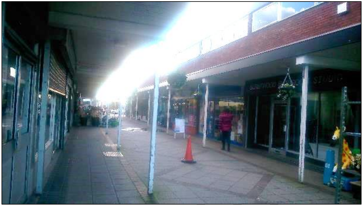
Local environment improvements are needed, such as within Burntwood Shopping Centre
